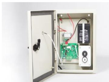
The **NECO DC Group Controller** can simultaneously operate up to 20 motors, making it the most efficient and cost effective fire safety product on the market.
