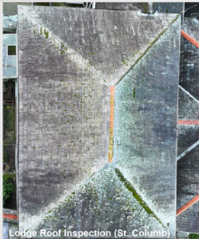
Lodge Roof Inspection (St. Columb)
