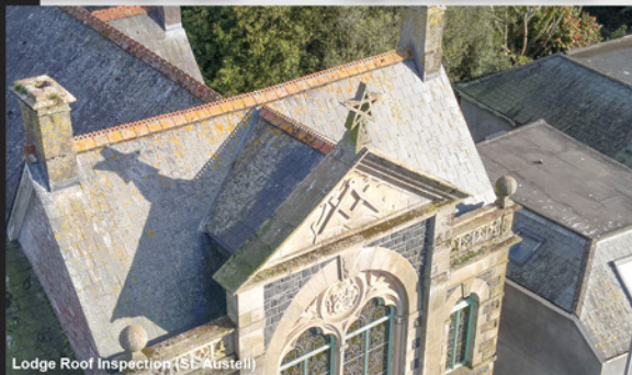
Lodge Roof Inspection (St. Austell)
