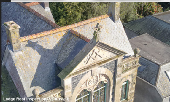
Lodge Roof Inspection (St. Austell)
