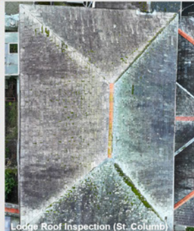
Lodge Roof Inspection (St. Columb)
