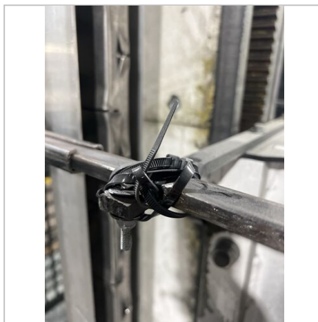
Operators fix for bad joint
